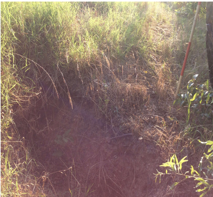
PHOTO 1 Description Abutment 1 right side slope 20' from end of bridge has 4' long 2' deep erosion area.
